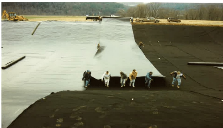
Installation of a lined manure pit in the Town of Candor, 1966
