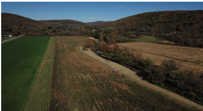
Berm removal site in Delaware County NY
