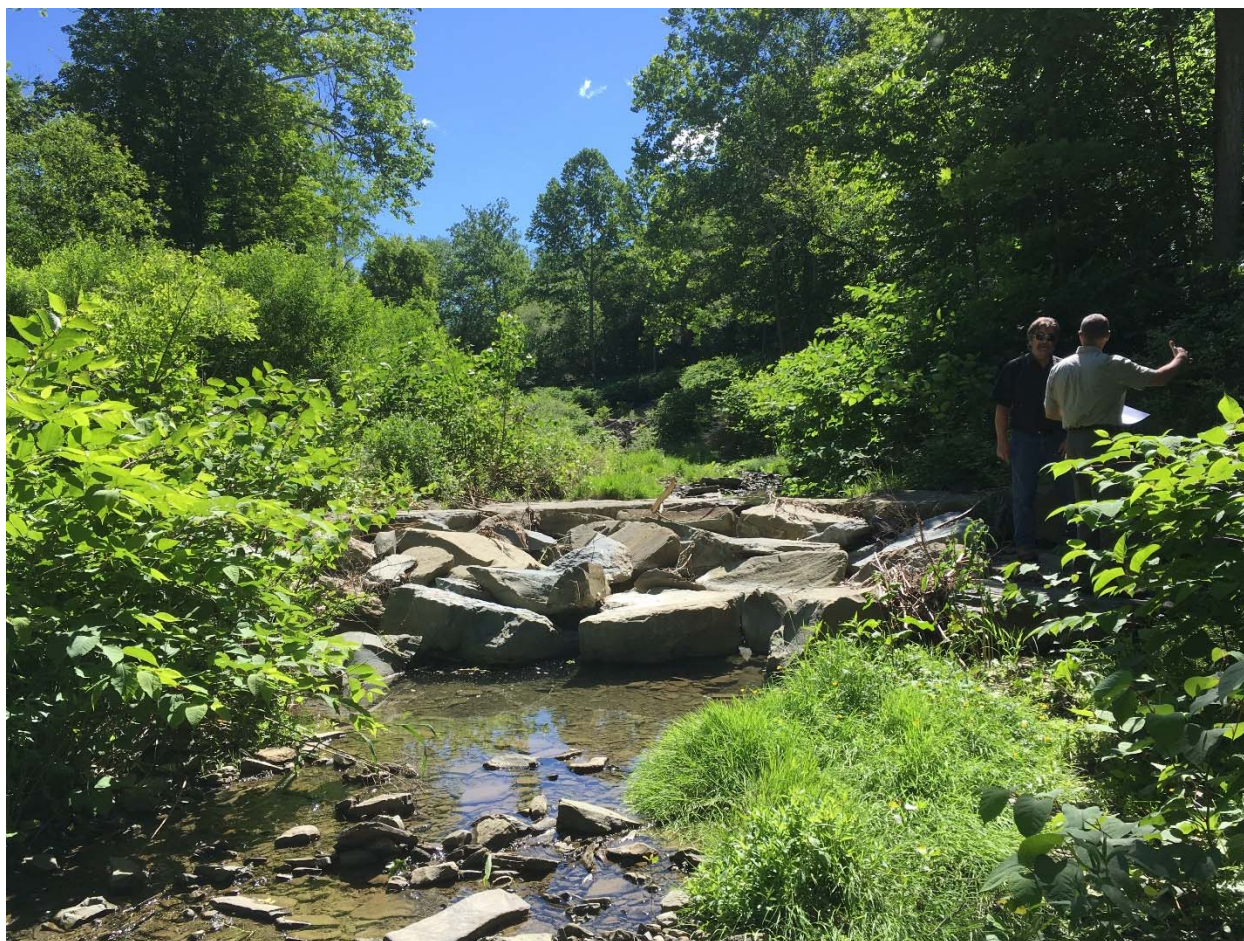
Figure 23. A portion of the NRCS grade control project at HT-3000. Note large boulders and lack of surface flow over the structure. Photo taken June 14, 2018.
