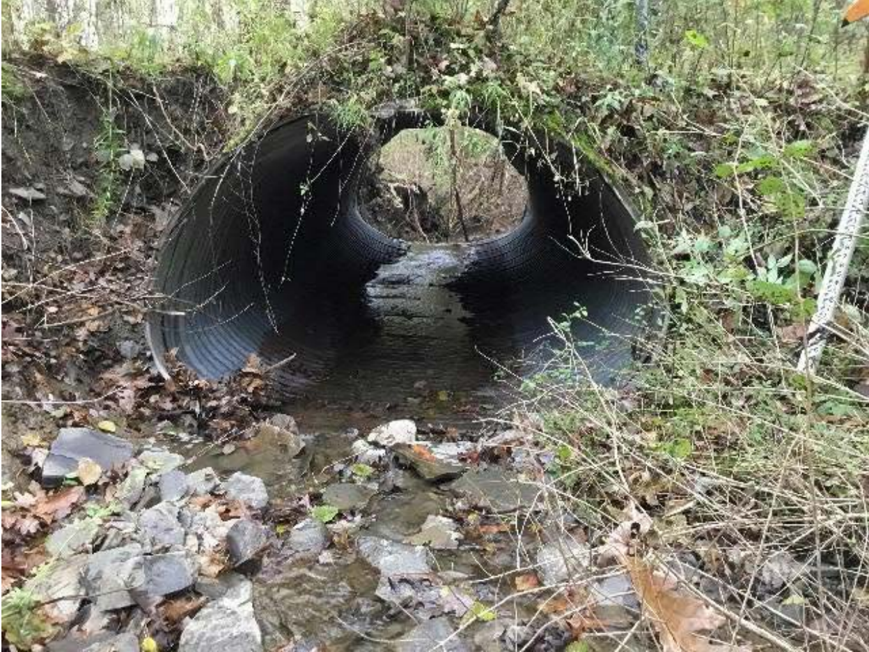
Figure 31. Private field access at Ht3-2700
