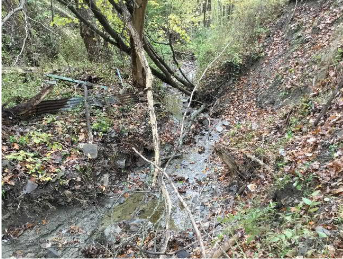
Carmichael Road over Tributary to Huntington Creek. Photograph of downstream channel. Note mass failure of slope on right bank.
