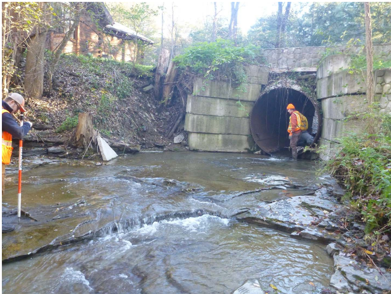
Figure 18. Looking upstream at culvert beneath private access at Ht-6100
