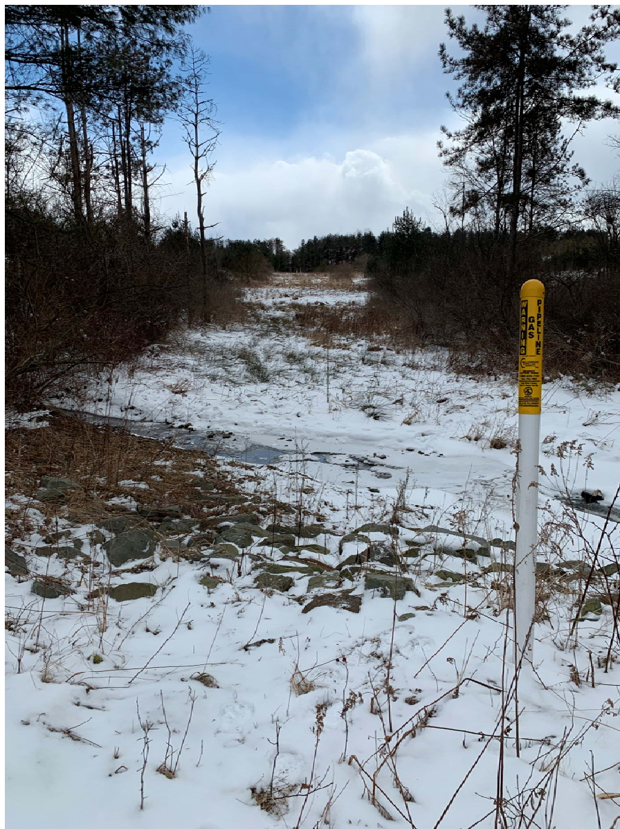
Figure 13. Broad floodplain at pipeline crossing at Ht-9600. Photo taken March 6, 2019.
