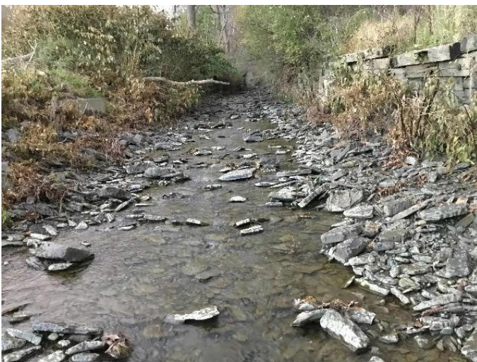
Huntington Creek channel upstream of Owego & Hartford Railroad bridge. Note leaning timber retaining wall lining stream channel on river left (right side of photo).
