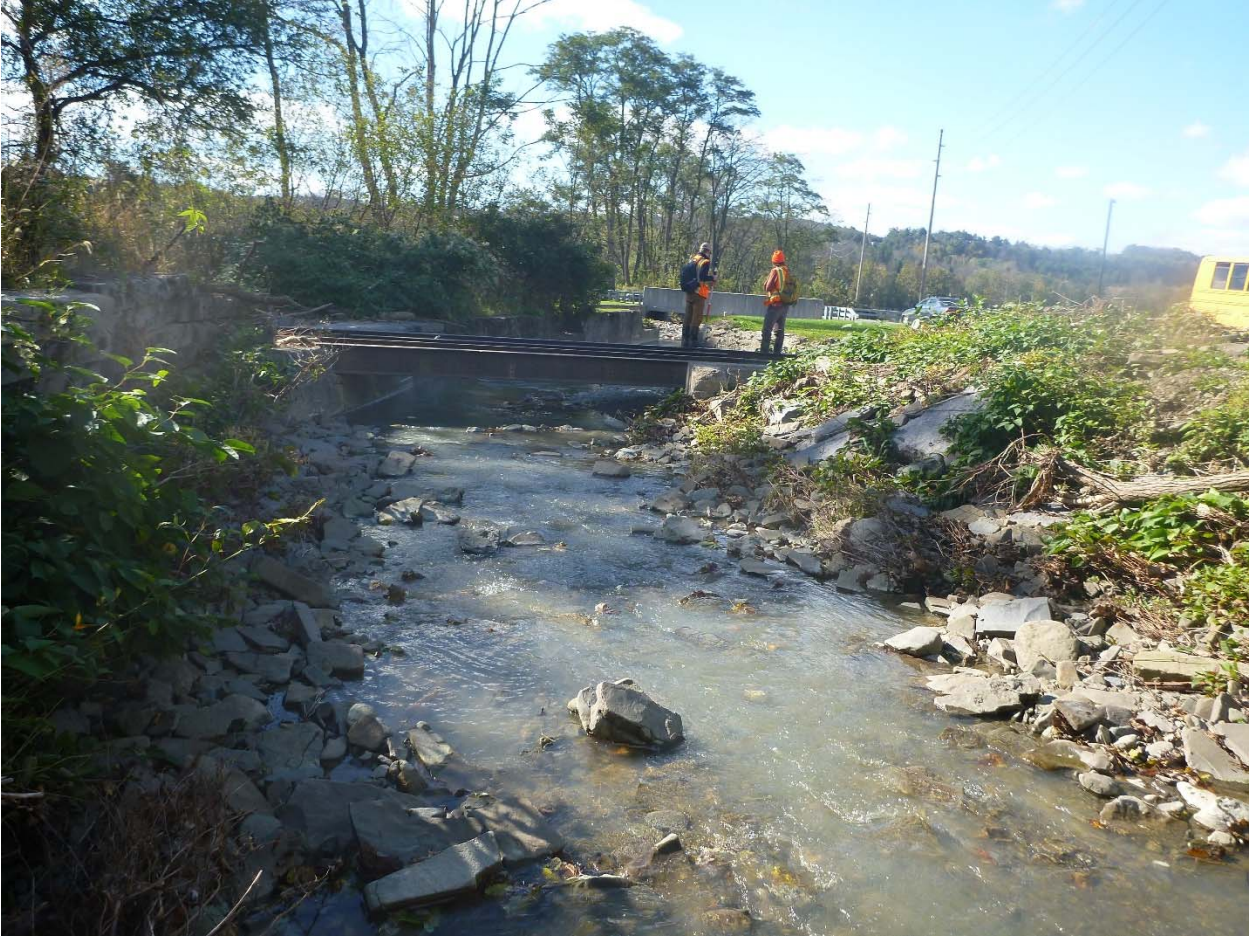
Figure 25. Looking downstream at the railroad crossing at Ht-1800
