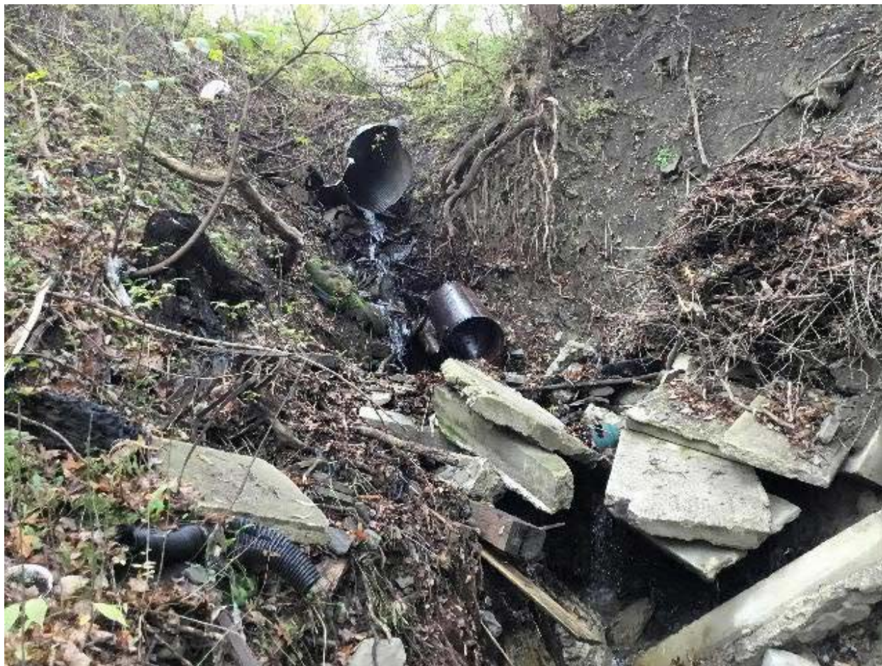
Figure 32. Carmichael Road culvert at Ht3-1900
