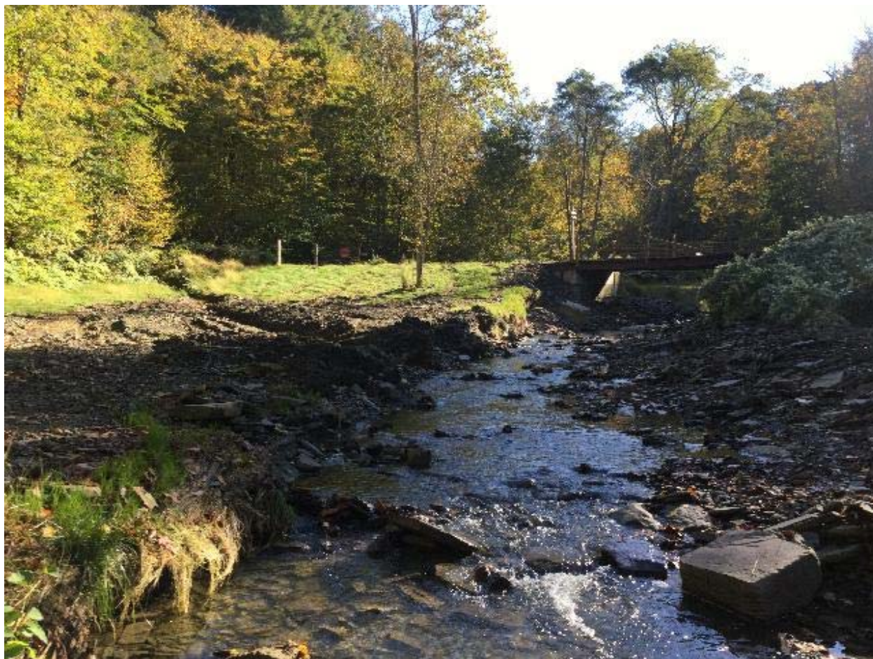
Figure 20. Looking upstream at cleared area around private access at Ht-4100. Note small drainage channel entering channel from river right (left side of photo).
