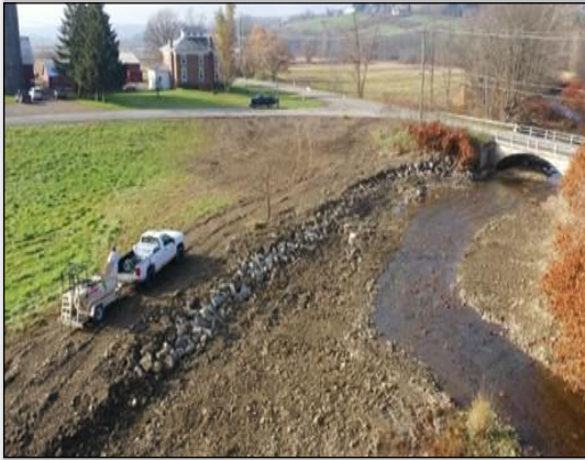
Streambank Protection Project in Cortland County (above)
