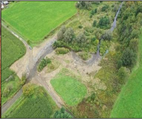
Streambank protection project in Otsego
